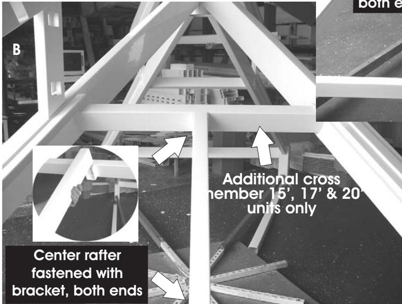
Fasten center rafters to brackets with screws and caps both ends.
