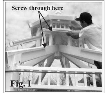
Hold roof panels in place with screw & cap through roof panel channels into roof panels (Fig. I)
